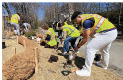
Erosion control in East Boston Greenway
